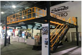
Example: A 25' x 25' mezzanine module used part-time in a Hayward factory and part-time at events like Autodesk University. This structure can be assembled or disassembled in just a few hours with 3 or 4 personnel.
